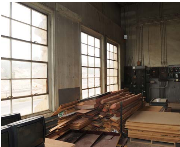
An interior view of the Laundry Building
