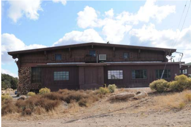
The existing west elevation of the Laundry Building
