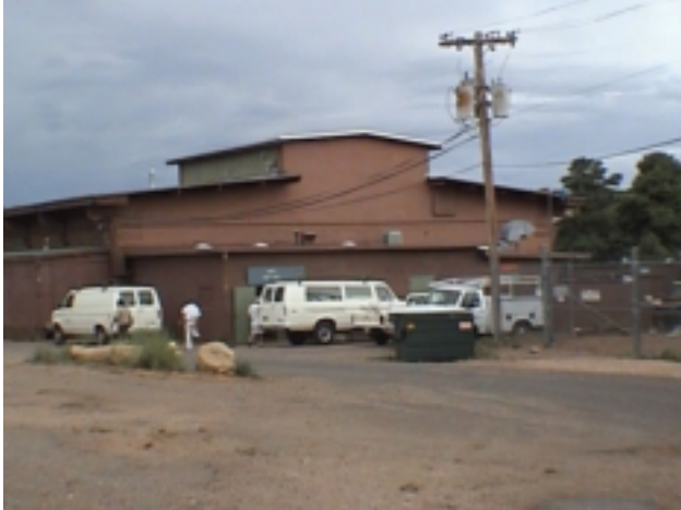
Photo of existing blank wall on east elevation
