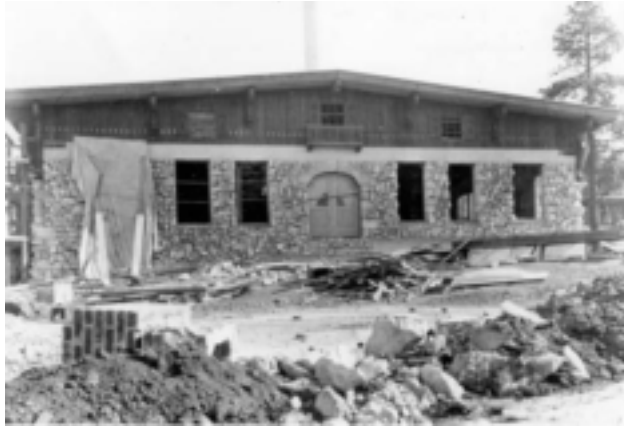
An historic Kolb Bros photograph of the Laundry Building under construction.
