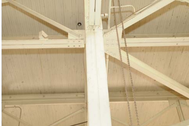
Photo of existing steel roof truss and column structure
