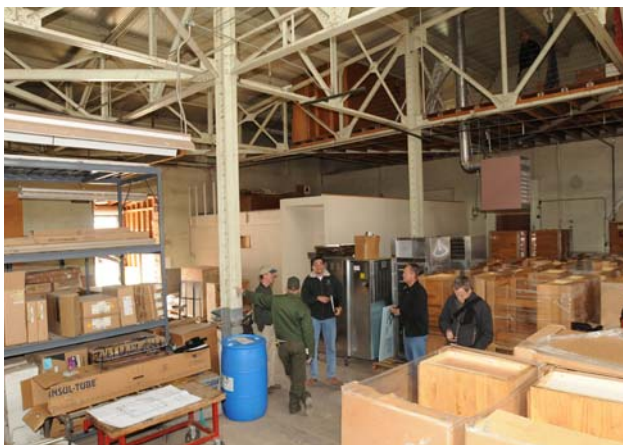
The existing interior of the Laundry Building with non-historic infill.
